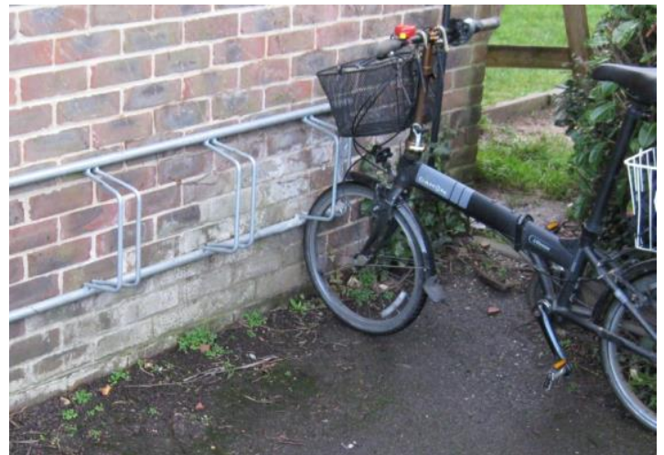
Figure 2: stands that only support the front wheel
