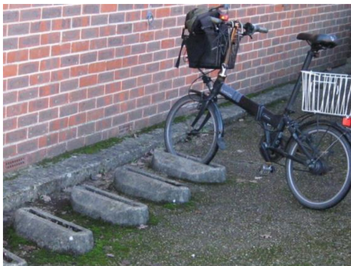
Figure 3: old concrete stands which only support the front wheel
