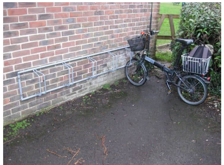
Figure 29: front wheel support stands in the car park of the Avenue Pavilion
